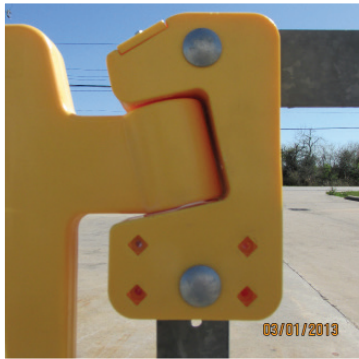
Hinge on angle iron guardrail
