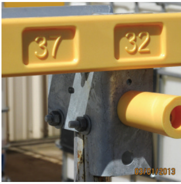
Block attached to pipe bracket
